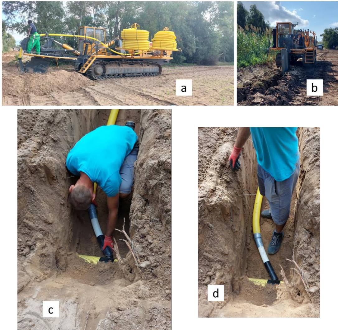
Figure 4. Some pictures of the operations for drain burying with an automatic drain-lying machine (pictures a and b) in one of the four farms in the Arborea case study, along with connections with the collector (pictures c and d)
