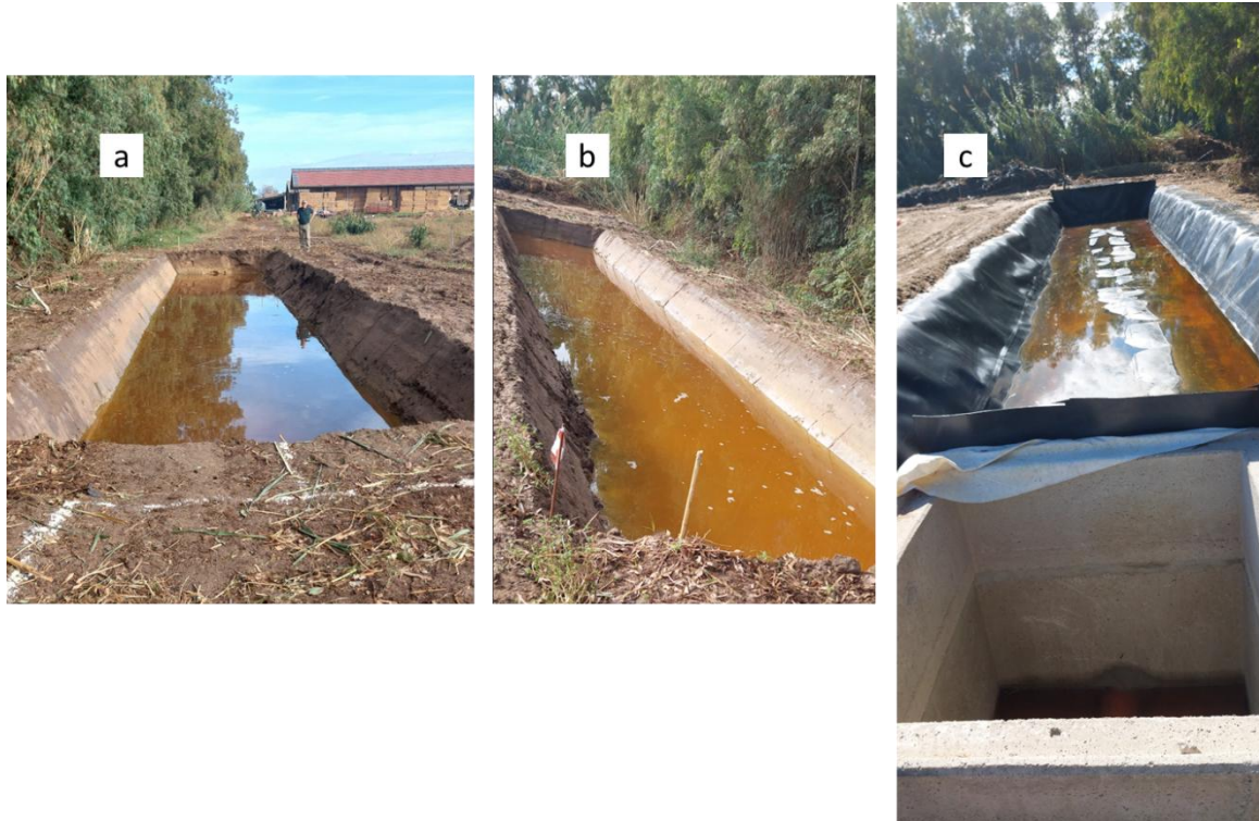
Figure 7. some pictures of the pit (pictures a and b) and its lining with the 2mm thick HDPE polyethylene waterproof membrane (picture c). The water in the pit comes from the shallow groundwater and has been pumped out before woodchip filling
