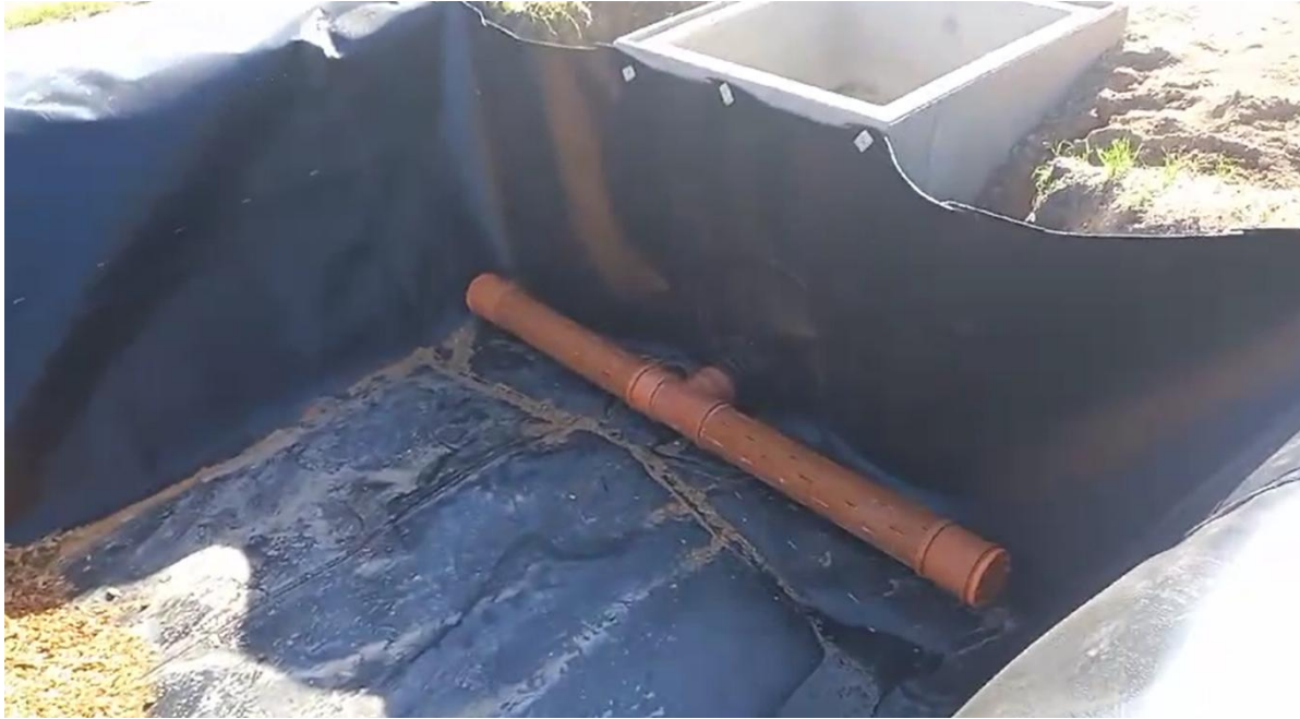
Figure 10. A picture of the transversal perforated PVC pipe diffusing the water to be treated over the whole width of the BR
