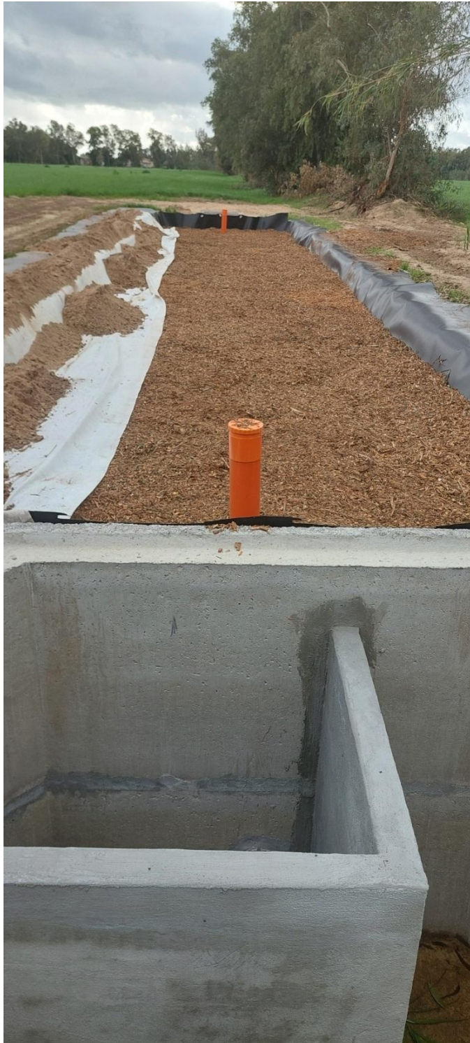
Figure 8. A picture of the woodchip filling the BR
