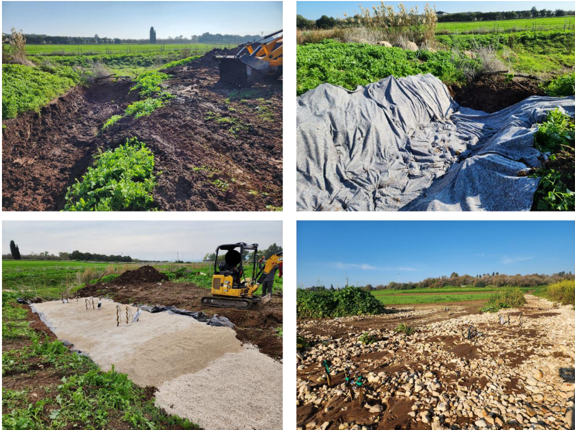
Figure 1. The bioreactor in Israel. From top left clockwise: the excavated pit for the bioreactor, lining the bioreactor internal wall, filling the bioreactor with the media and, finally, covering with soil
