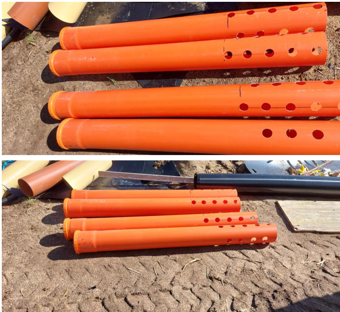
Figure 11. A picture showing piezometer installation along the BR
