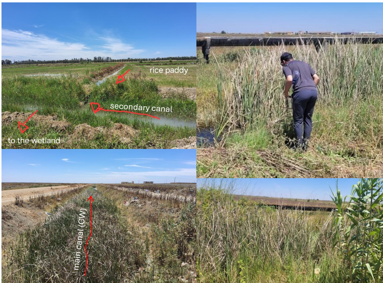
Figure 6. The CW at the Sidi Allal Tazi Experimental Farm. The arrows indicate the path of the surface drainage water. The two figures on the right provides a detail of the vegetation mainly existing in the CW (see the text)
