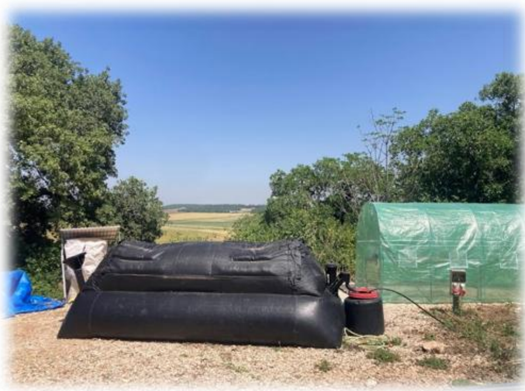
Figure 1. Farm farm-scale anaerobic digestion system in Newe-Ya'ar Research Center, Israel
